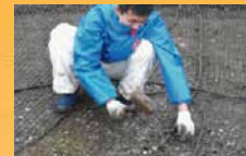
生物付着除去作業 (Elimination of sessile organisms)
